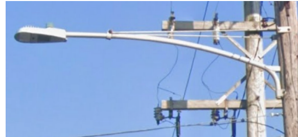
Cobra-head style light fixture
